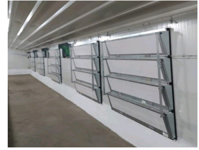
Tunnel inlet system mt system
