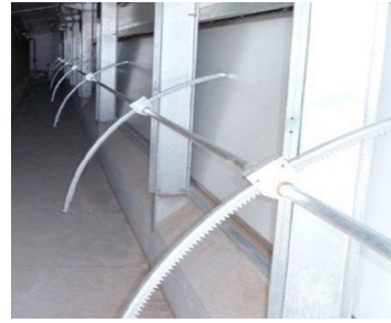
Tunnel inlet w/rack&pinion system
