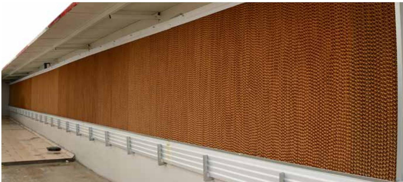
**PAD COOLING SYSTEM WITH INTEGRATED WATER SUPPLY**
